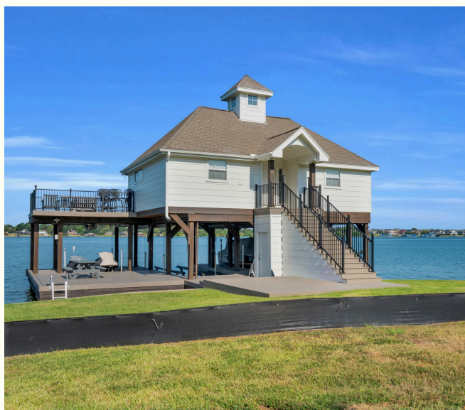
Lake Conroe Dr, boathouse on pilings.
